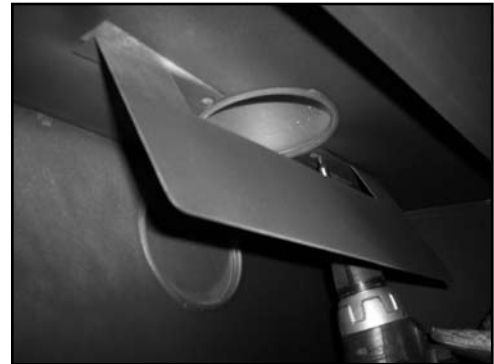
Figure 7.7b Remove Flue Visor
