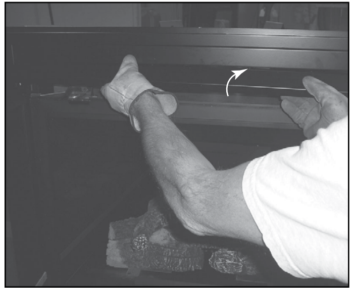
Figure 15.10 Installing Hood
