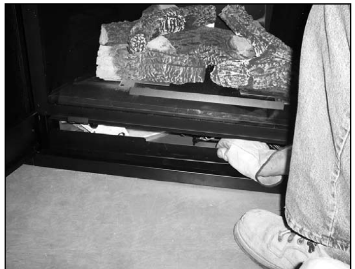
Figure 15.11 Installing Floor Cover
