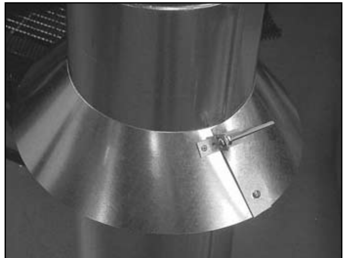
Figure 10.17 Assembling the Storm Collar Around the Pipe
