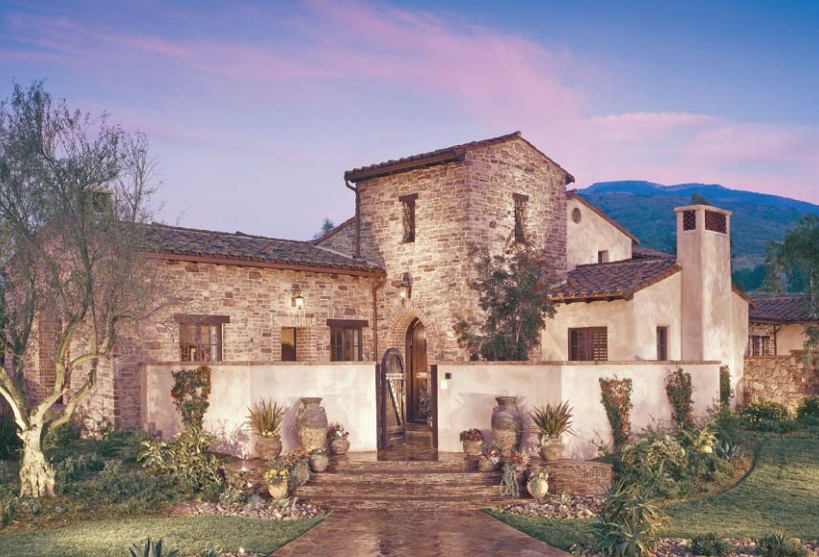
Orchard Cypress Ridge with an overgrout technique
