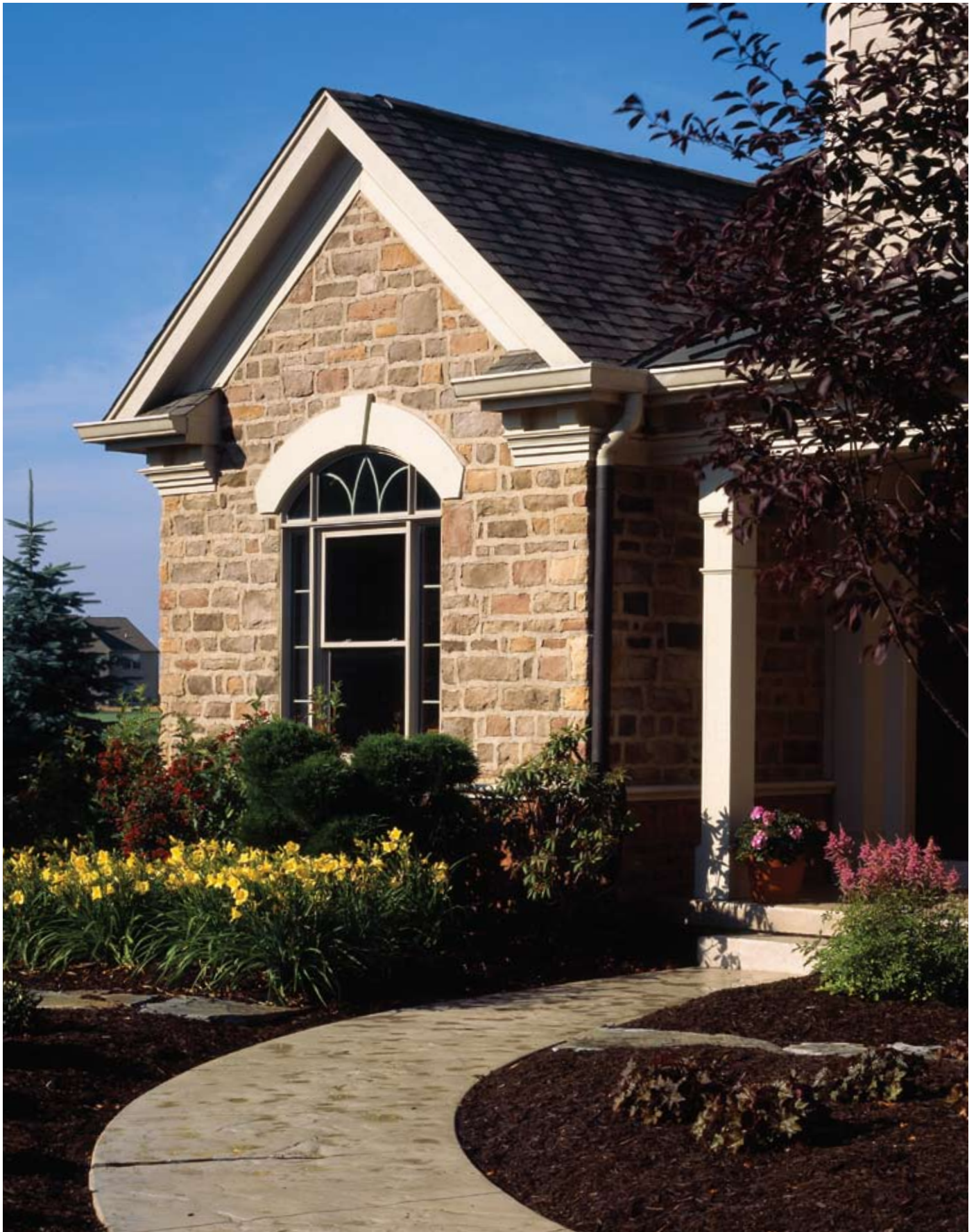
Bridgeport Limestone with an overgrout technique
