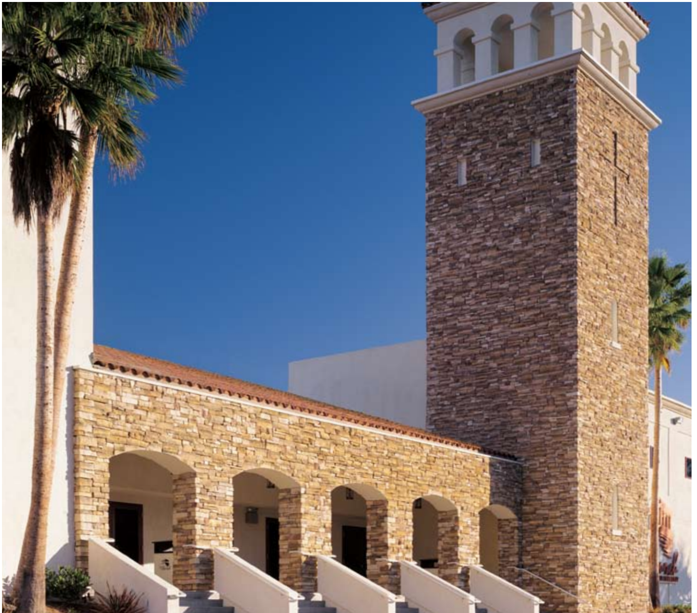
Western Wisconsin Weather Edge with a dry-stack grout technique
