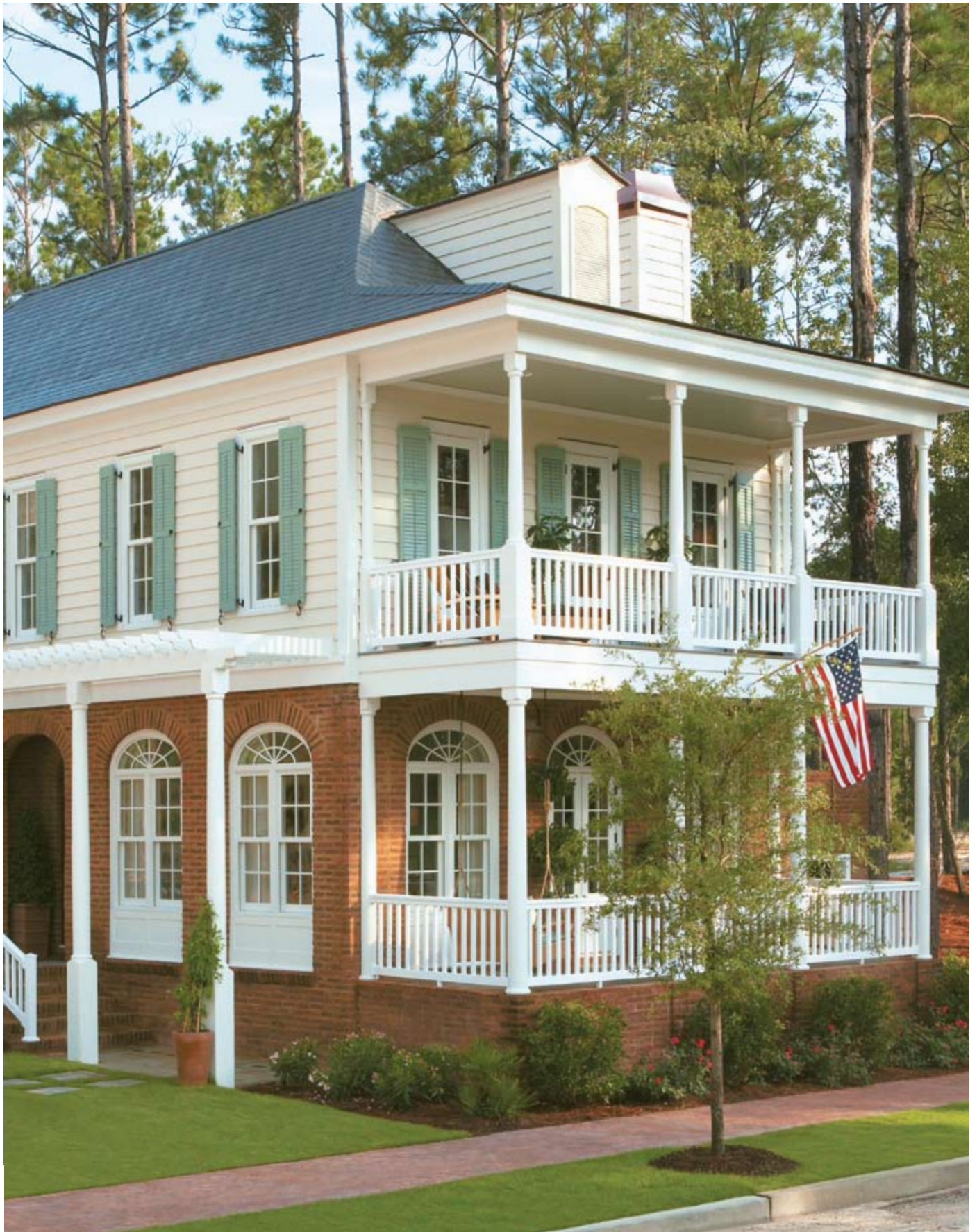
Bracciano RomaBrick with an overgrout technique
