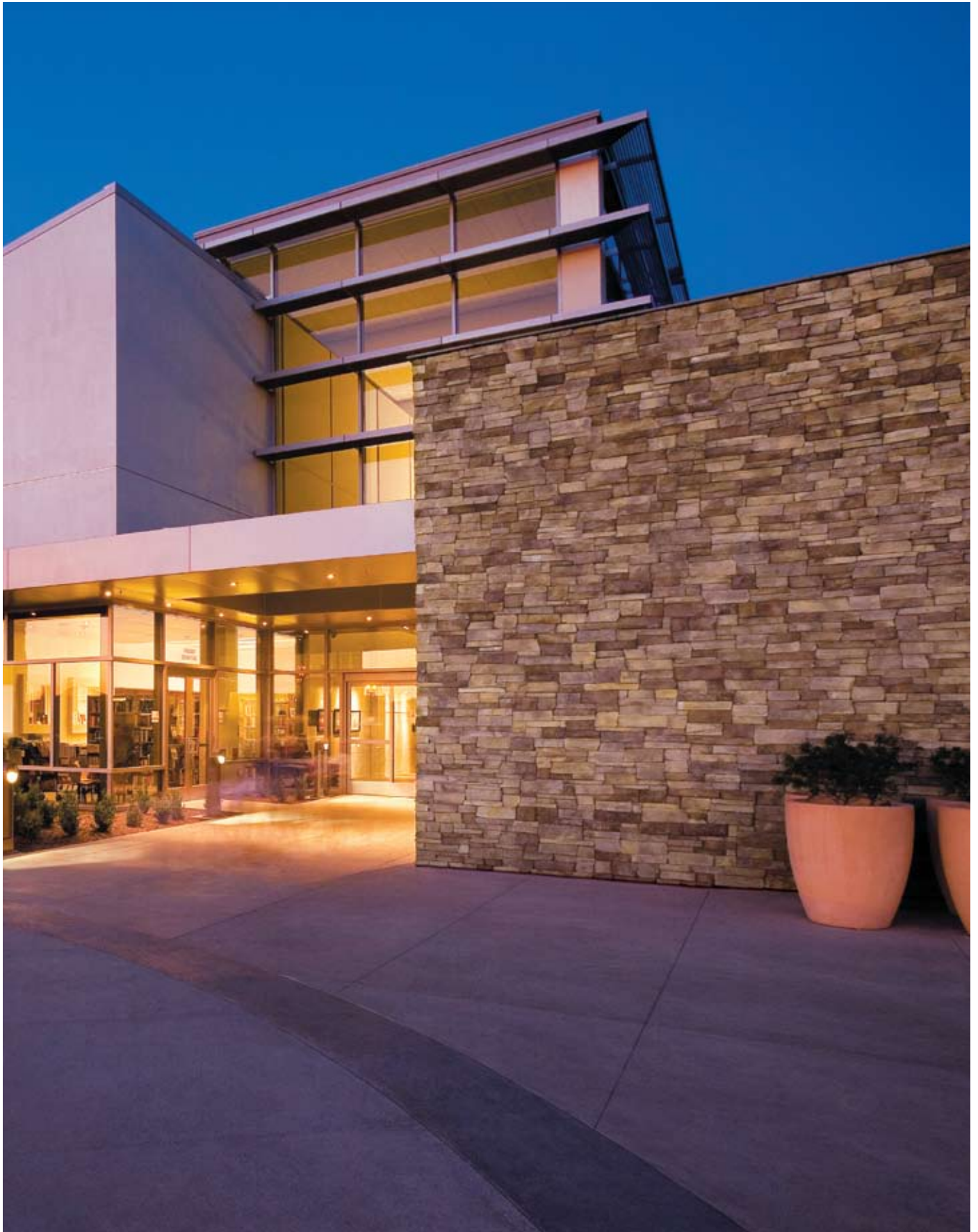
Manzanita Cliffstone with a dry-stack grout technique
